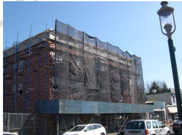
Building under renovation at W. Fairview and Irvington
