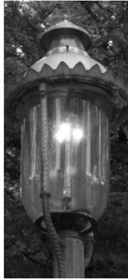
Three glowing mantles are visible inside the globe of this gas lamp. If they're not all glowing in a lamp near you, please contact PSE&G.
